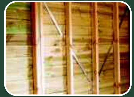
Standard 2.1m high walls with steel bracing
